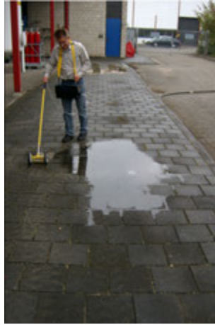
FIGURE 3.3 Leak searching using ‘sniffing’ equipment - image courtesy of KIWA
